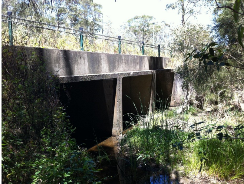
Figure 4-1 Southern Catchment Culvert
