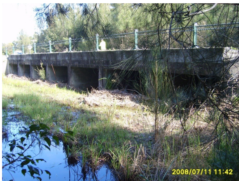
Figure 4-4 Northern Catchment Culvert (source: Great Lakes Council)
