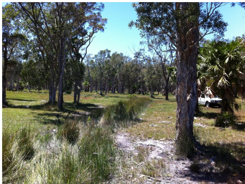
Figure 4-2 Typical Drainage Swale
